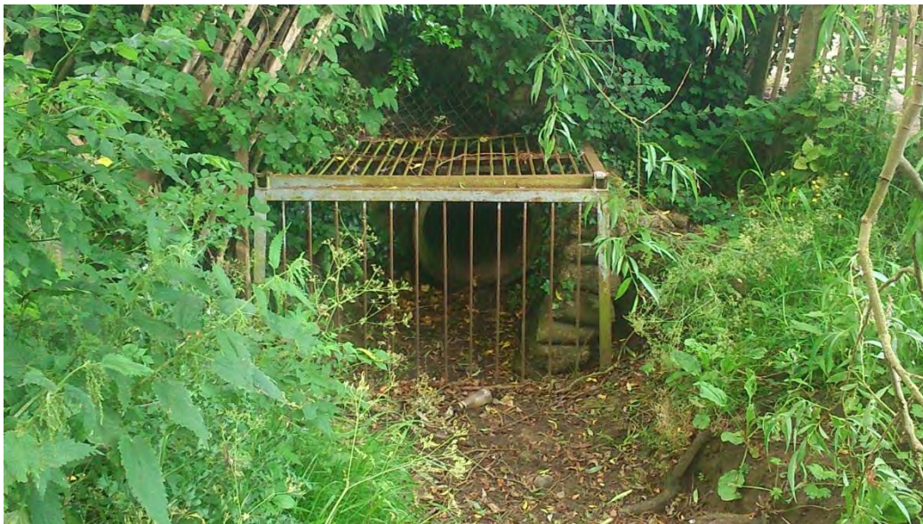
Figure 5-3 Culvert inlet behind no. 38 Damian Way
