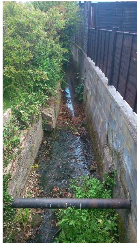
Figure 5-5 Southern watercourse on Damian Way
