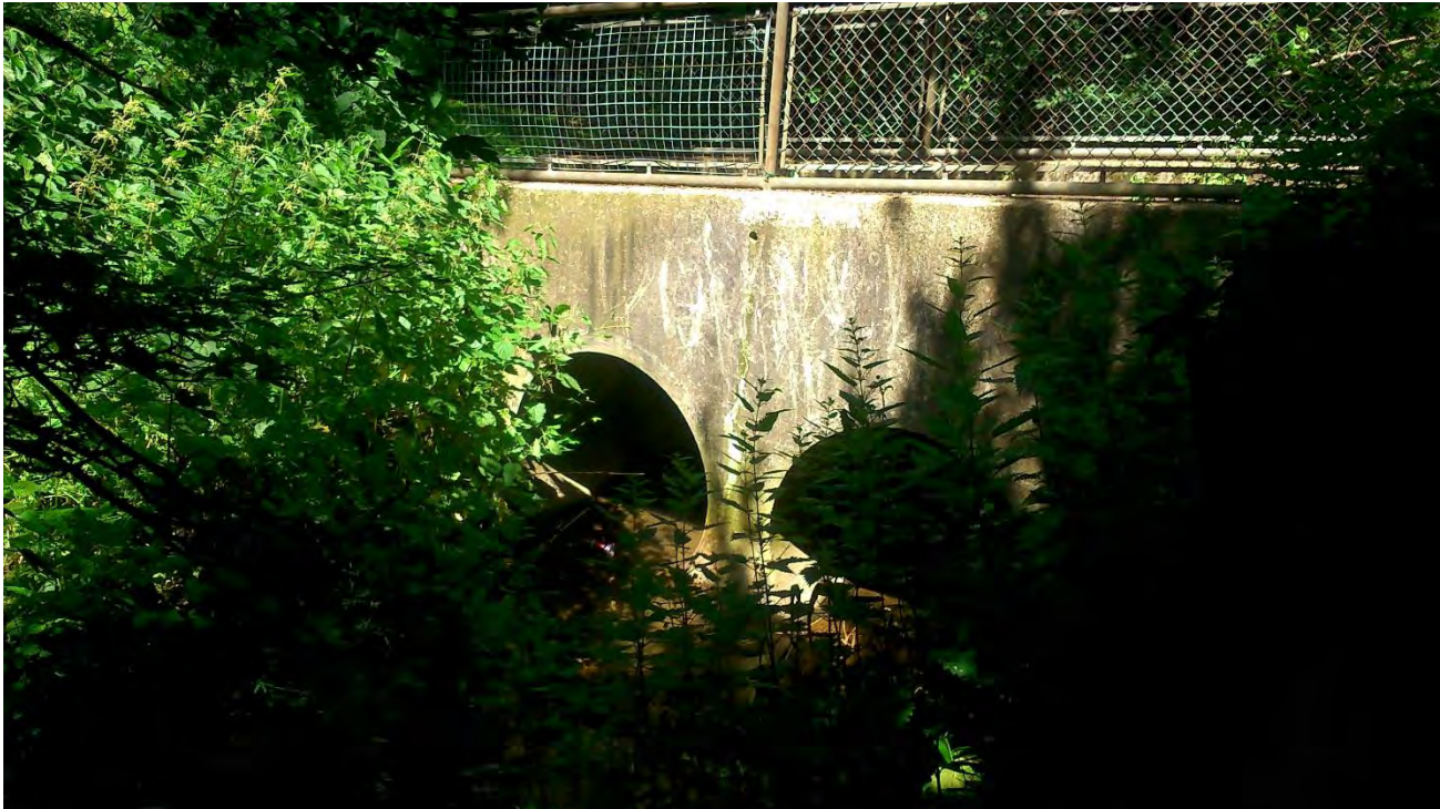
Figure 5-1 Culvert under footbridge on Herring Stream
