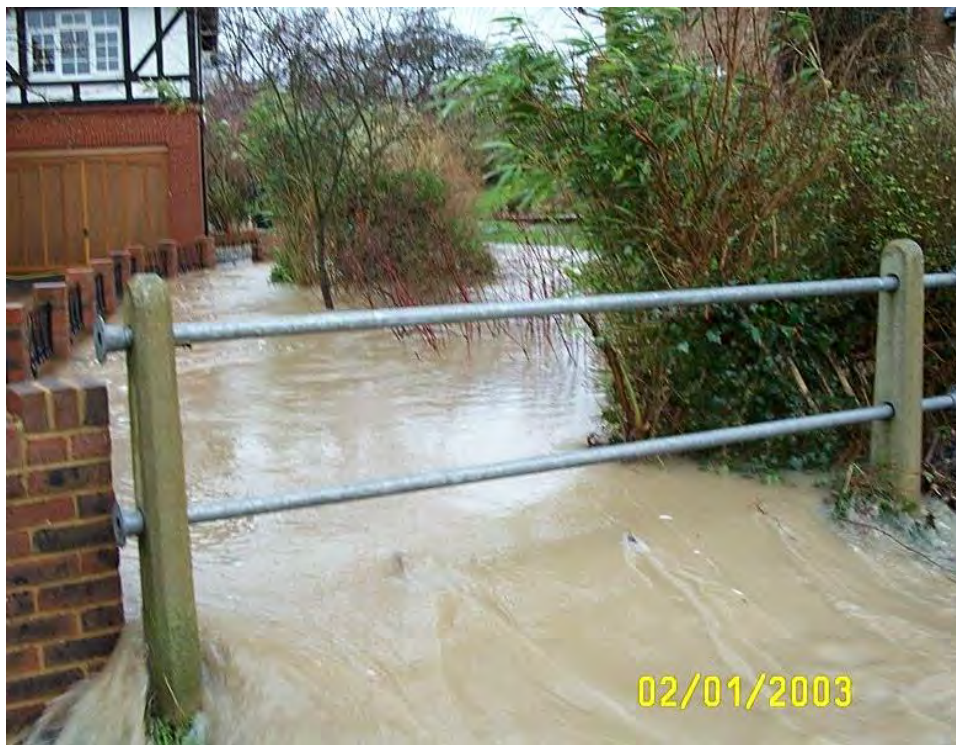
Figure 4-2 Flooding at the Lodge Lane culvert in 2003
