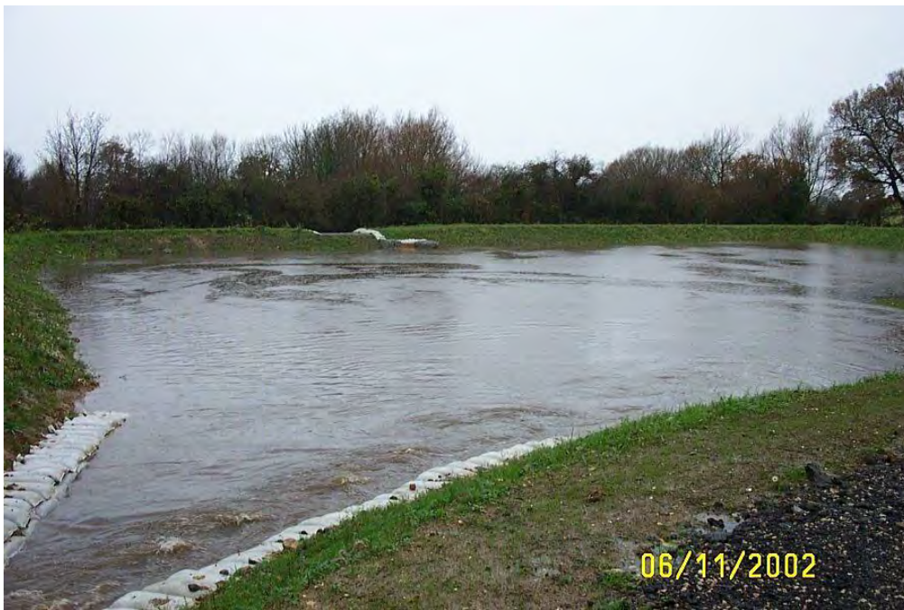
Figure 2-2 Damian way balancing pond during a storm event in November 2002
